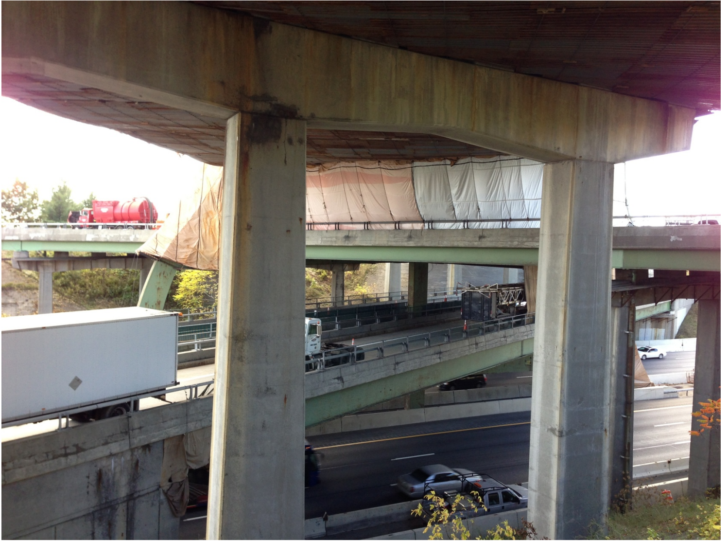
Upper Level 4 – Cable Supported/Metal Deck Platform System Level 3 – Containment To Roadway Supporting Arch Containment – Left
