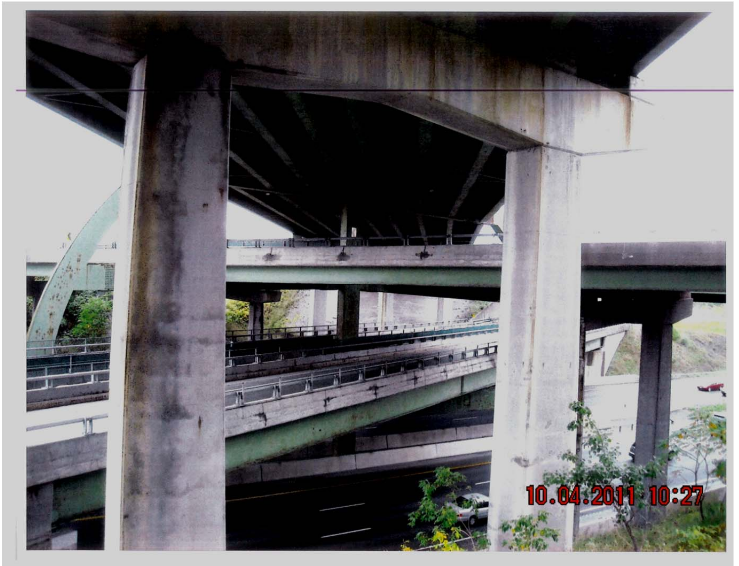
Steel Arch Supported Lark Dove Arterial – Albany, New York
