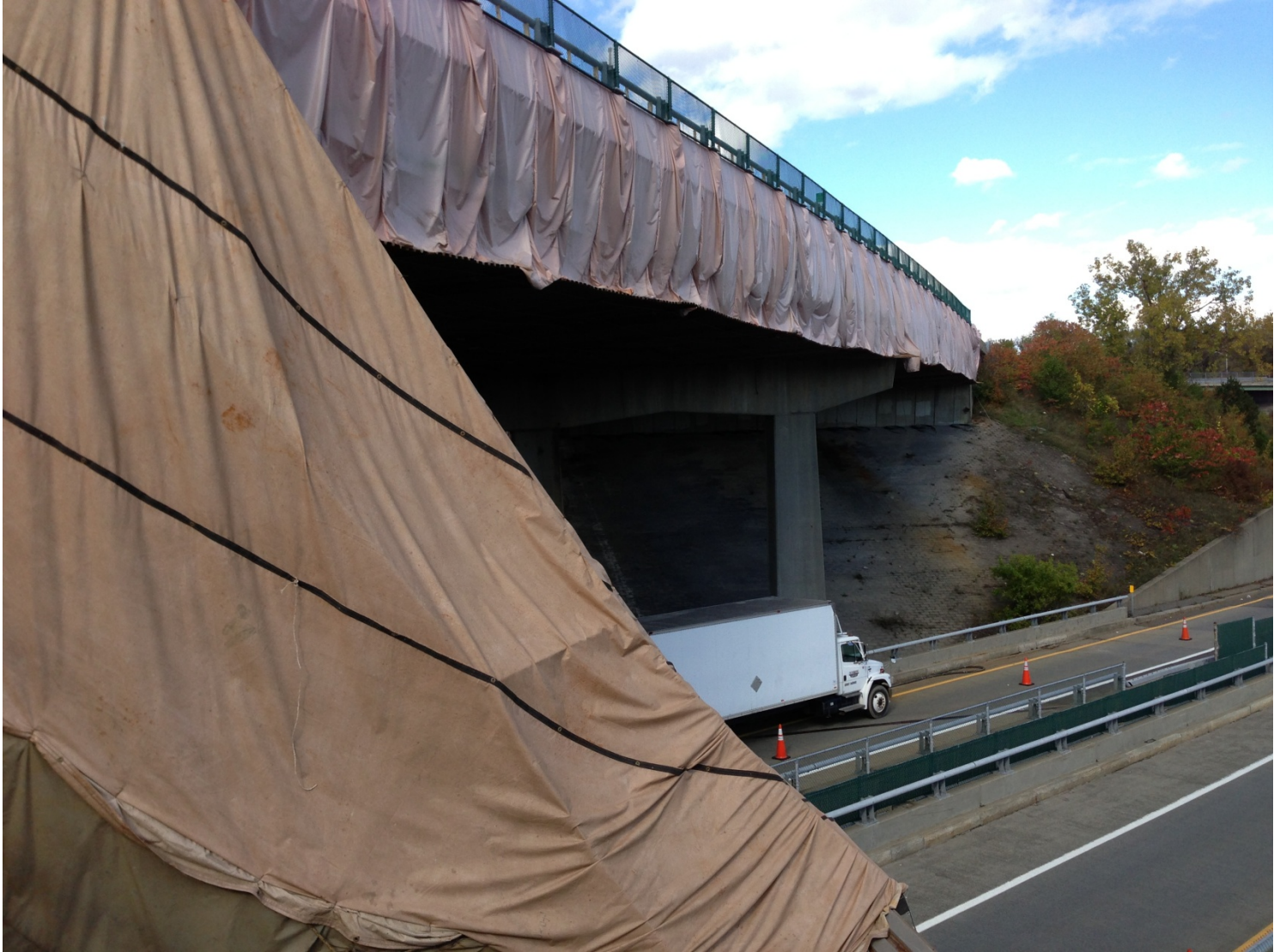
Cable Supported/Metal Deck Platform & Containment – Upper Level 4 - Right Supporting Arch Containment - Left
