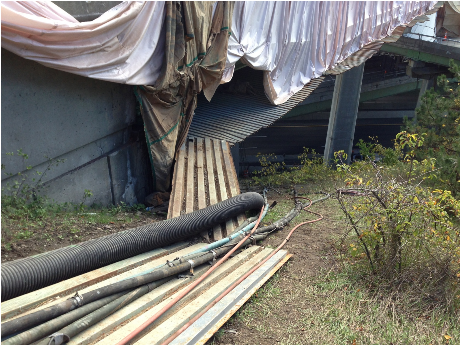
Cable Supported/Metal Deck Platform & Containment – Upper Level 4
