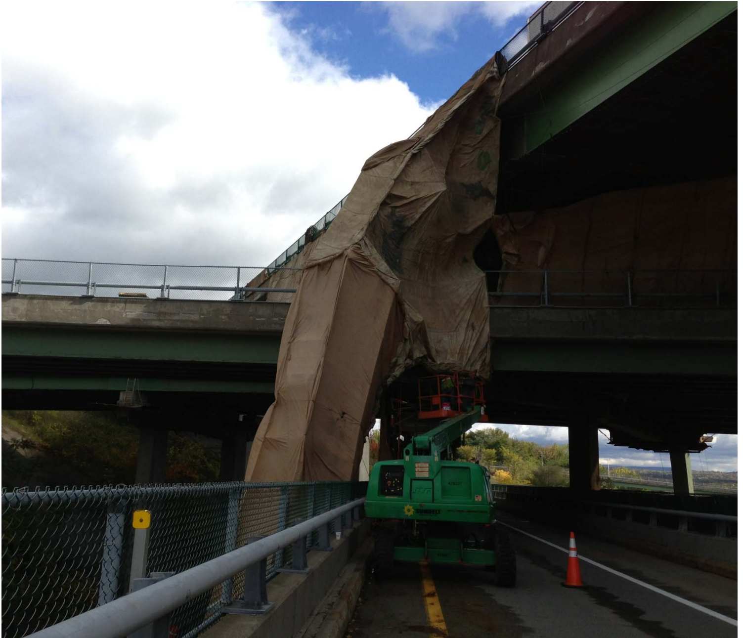
Level 3 – Containment to Roadway Supporting Arch Containment - Left
