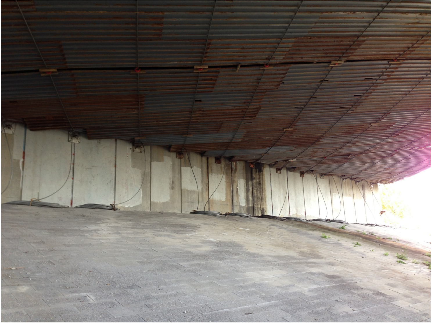
Anchor Plate End Assemblies – North Abutment
