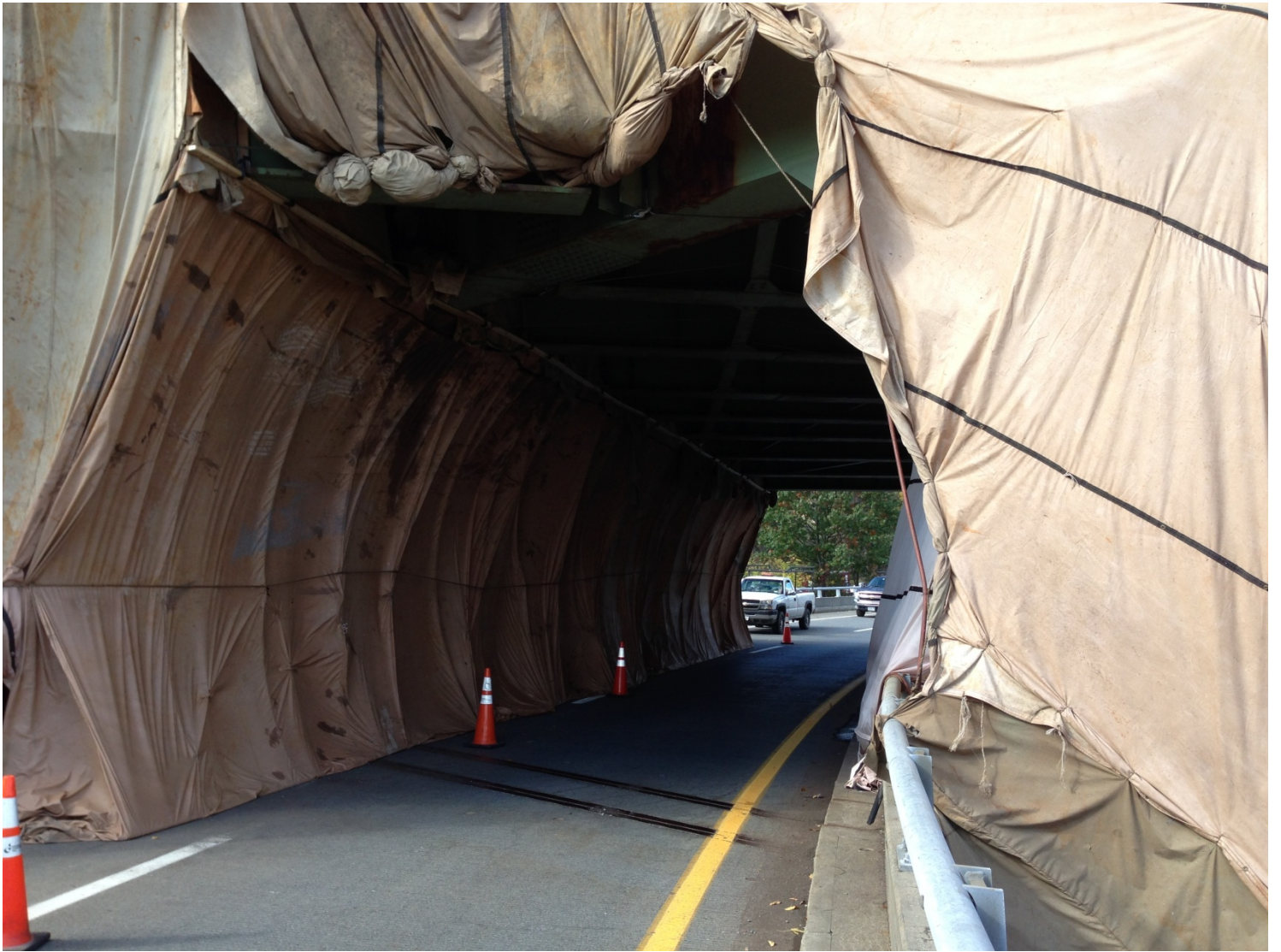
Upper Level – Containment to Roadway
