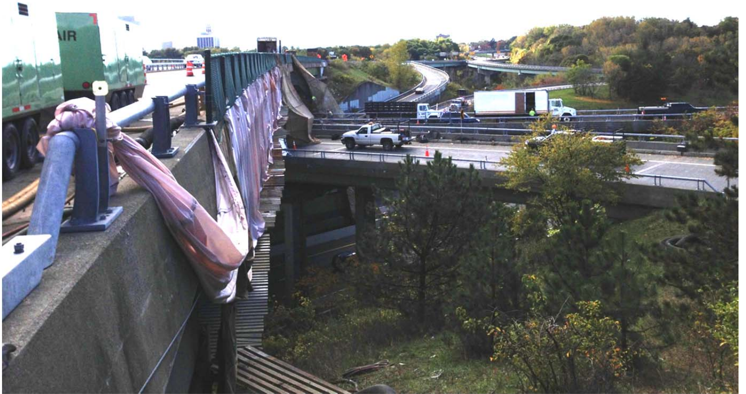
Cable Supported/Metal Deck Platform – Upper Level 4
