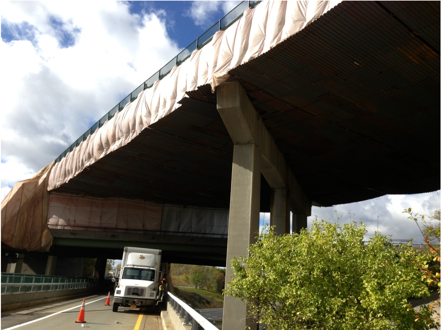
Upper Level 4 – Cable Supported/Metal Deck Platform System Level 3 – Containment To Roadway
